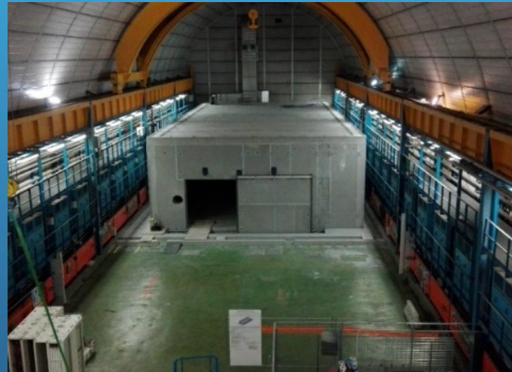
Concrete bunker during construction
