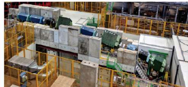
September 19, 2018 – HV @ 180 kV ready for beam!
