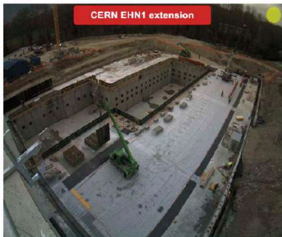
March 2016, construction of EHN1 extension
