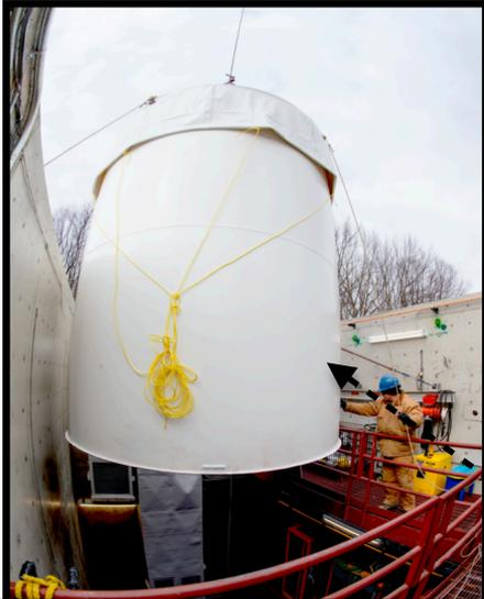
Steel tank holds 26-ton of Gd-loaded water
