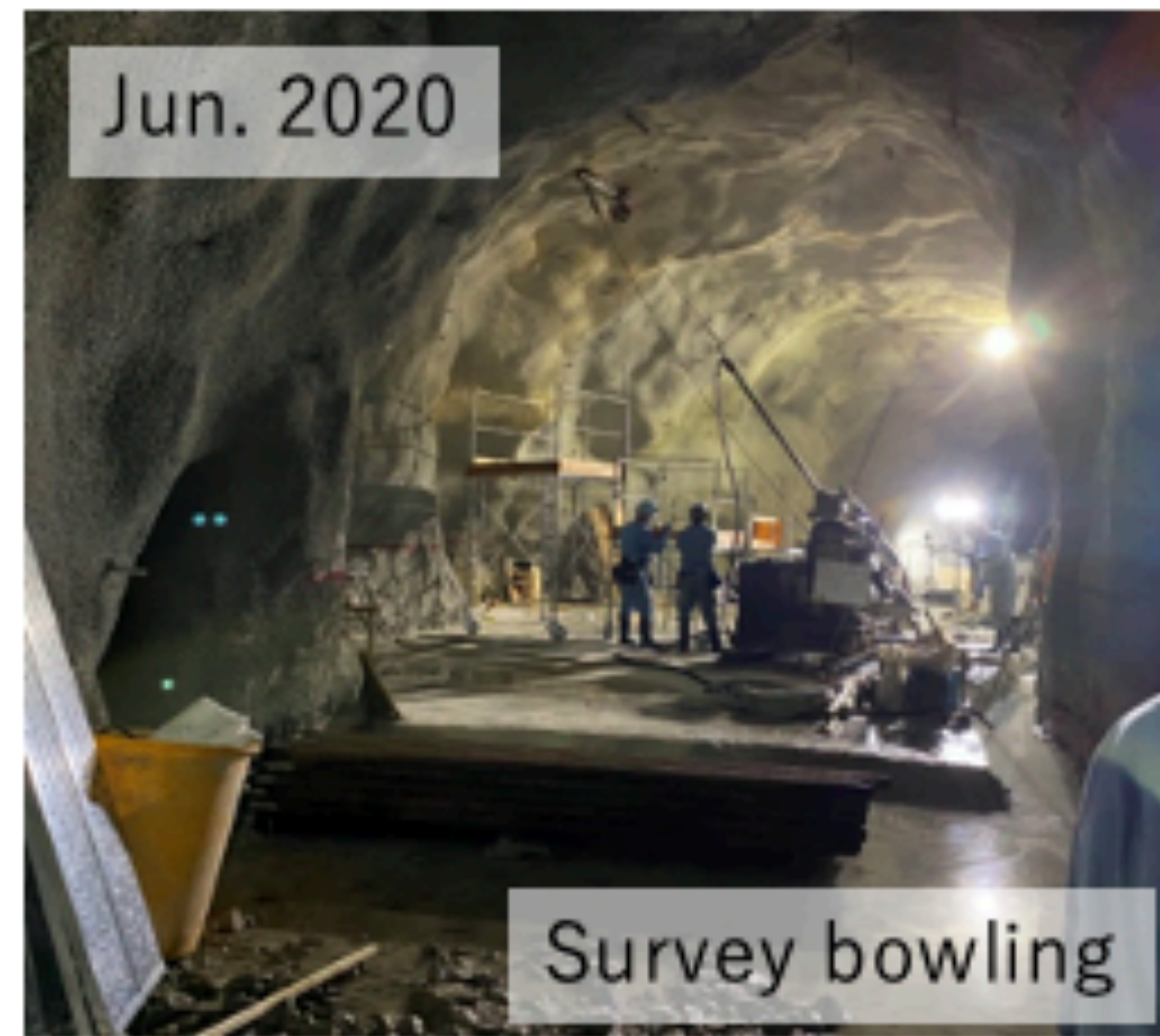
Survey tunnel Near the center of the (future) HK dome
