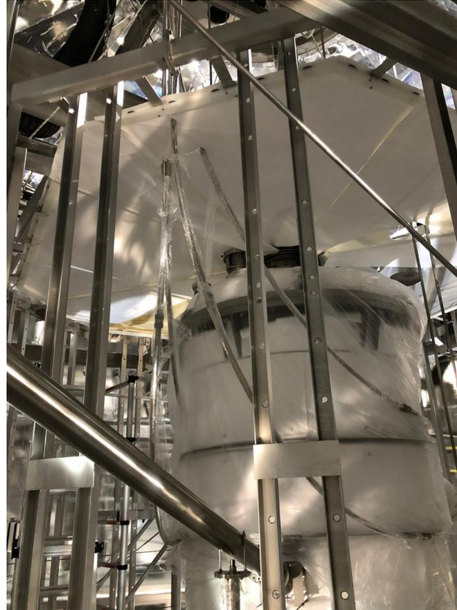
Wrapping of Neutron Generator beam holder and pipe
