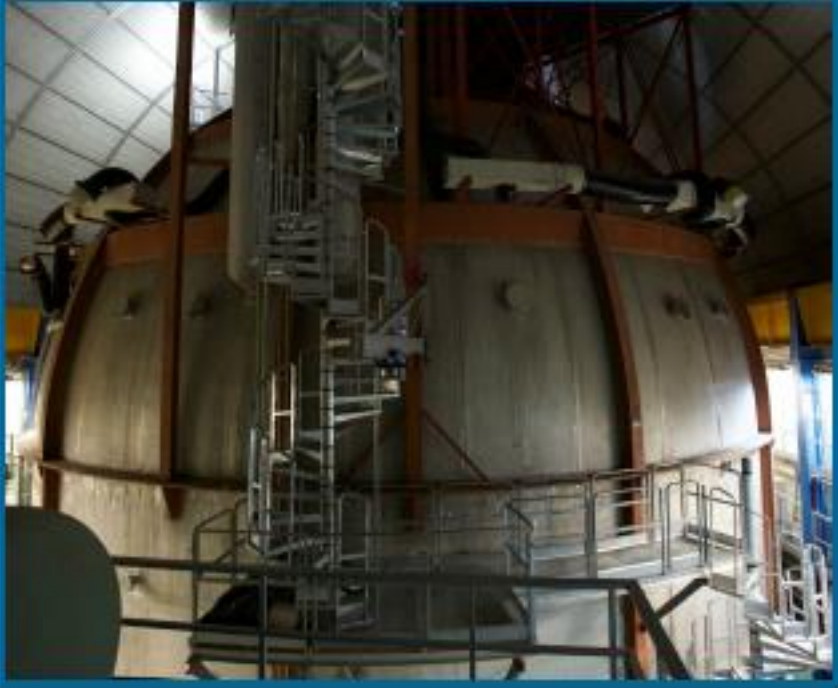
Before thermal insulation
