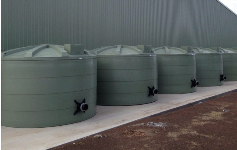
Reference tank size – 3.9m diam., 2.5m deep
