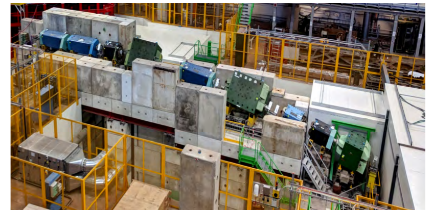
September 19, 2018 - ready for beam!
