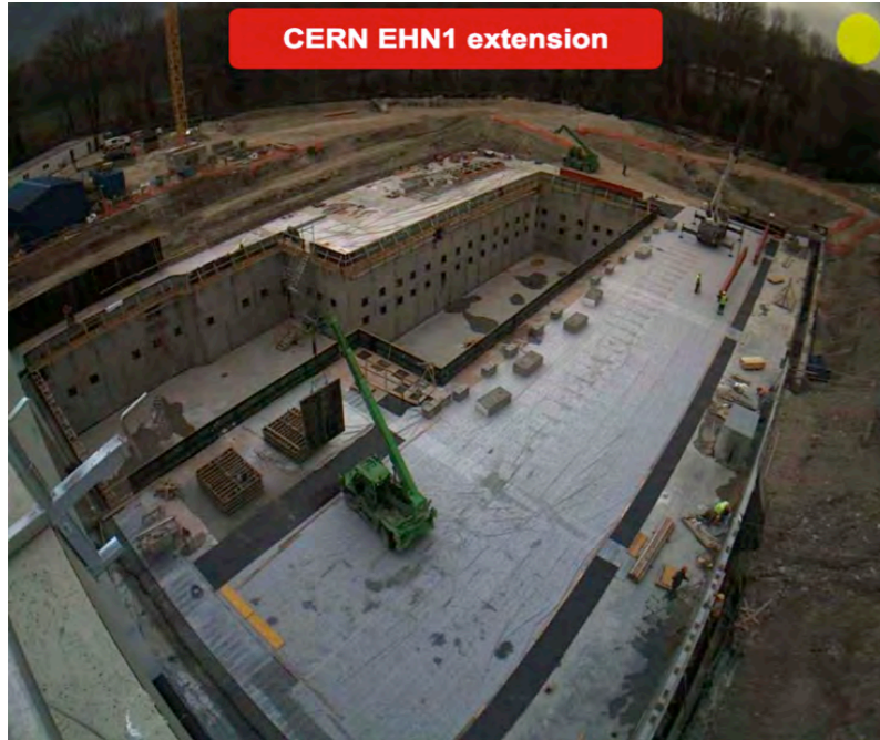
March 2016, construction of EHN1 extension
