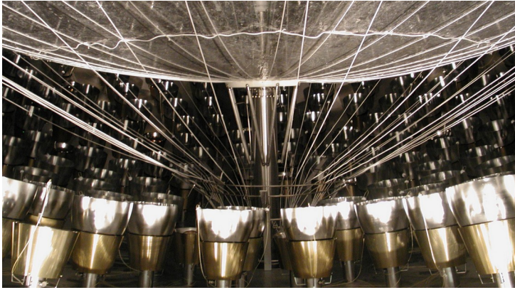
During the construction
