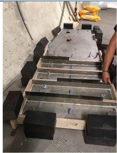
Survey and positioning of baseplates for muon filters
