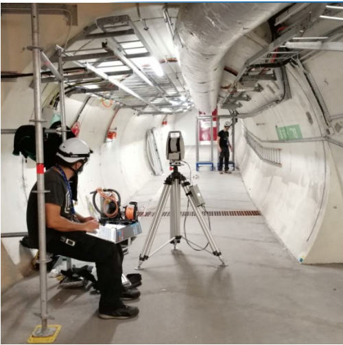
Survey and positioning of baseplates for muon filters
