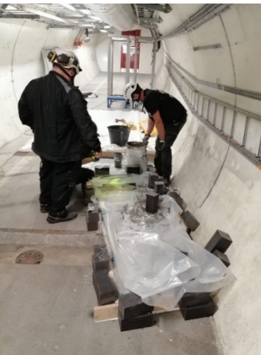
Formworks and grouting of baseplates
