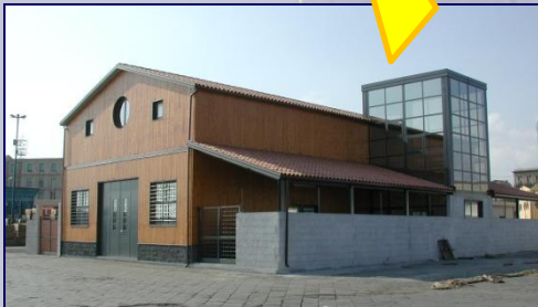
LNS Test Site Laboratory at the port of Catania
