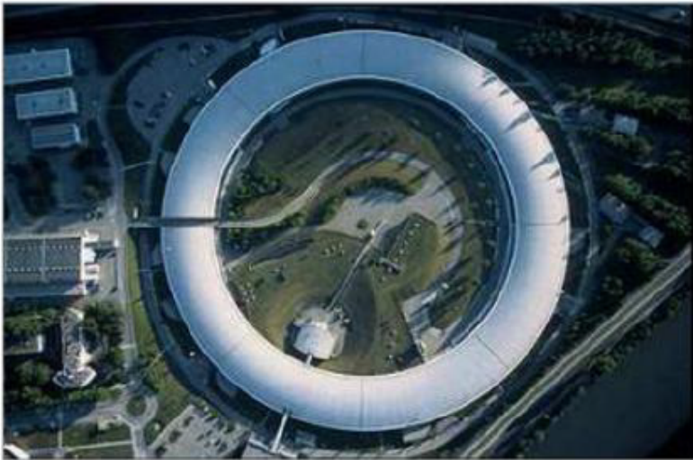
Aerial view of the ESRF (courtesy of ESRF/D. Morel)
