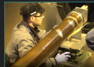
Removing the beam pipe
