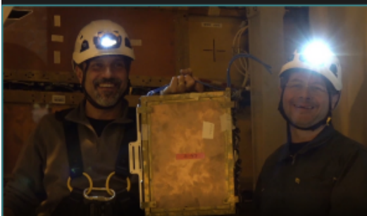
Dismantling of M1 muon station
