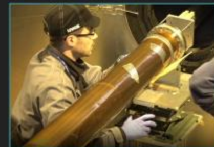
Removing the beam pipe
