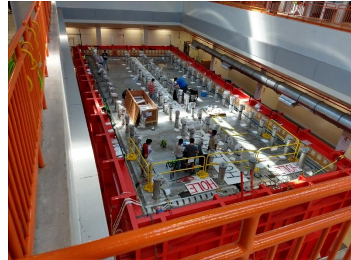
Chimneys installation (October 2018)
