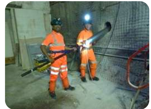
Bore hole detector installation
