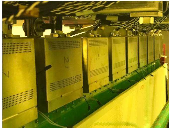
Installed CE boxes
