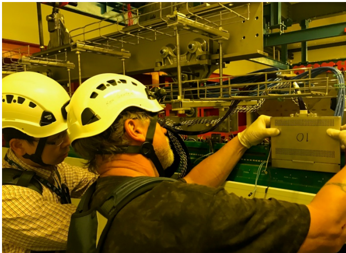
CE boxes installation on APA
