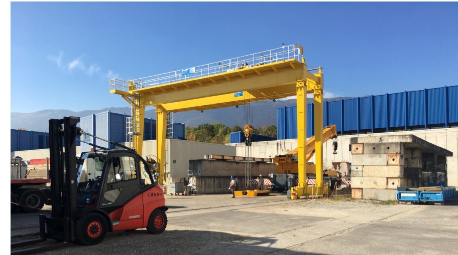
Preparation CR0 area (O2 Data Centre)
