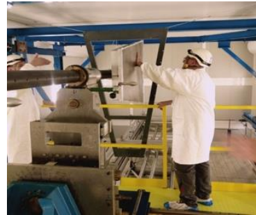
Install new ROC
