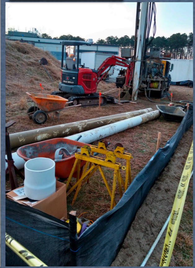
Wells digging and pipe installing
