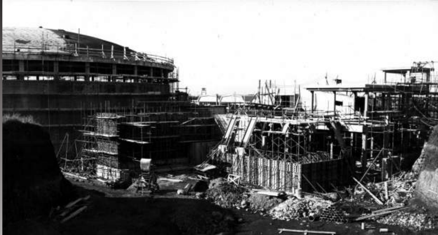
Construction of the pion hall (later BTF), 1966
