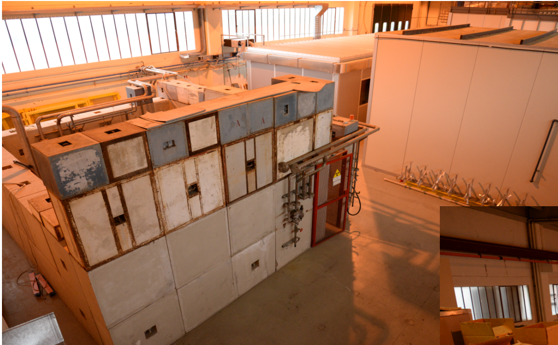
LNF building #7: the old bunker
