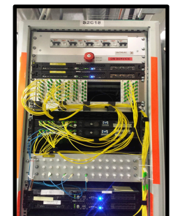
Rack in Service Cavern (USC) 70 m underground
