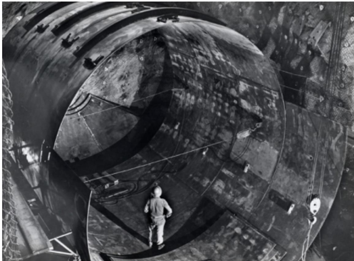
1965: Ray Davis inside chlorine tank used for solar neutrino detection
