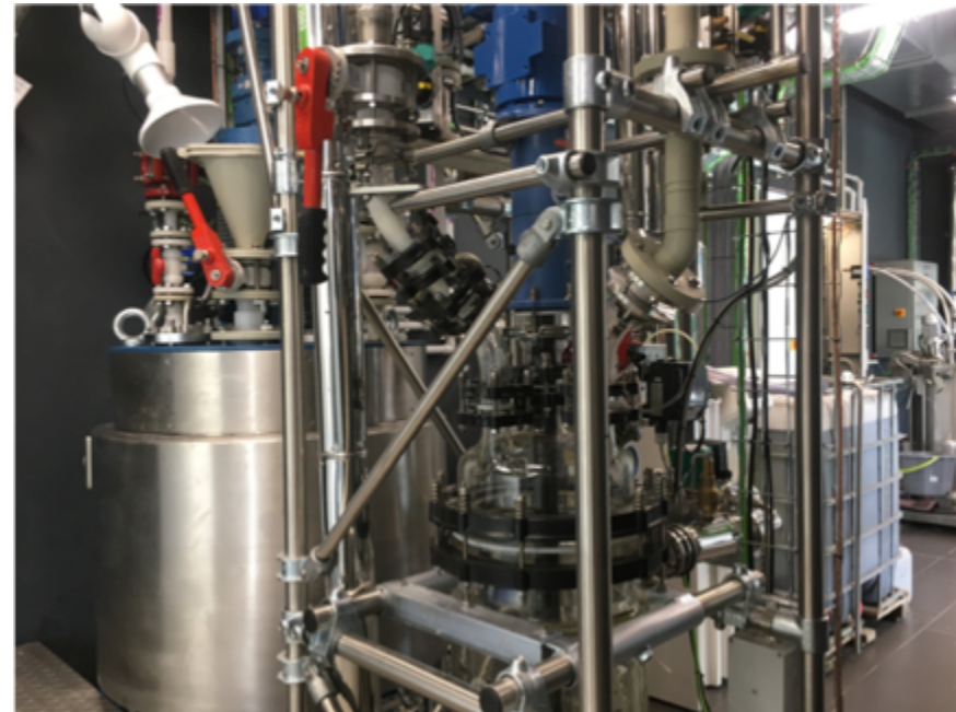
GO Pilot plant
