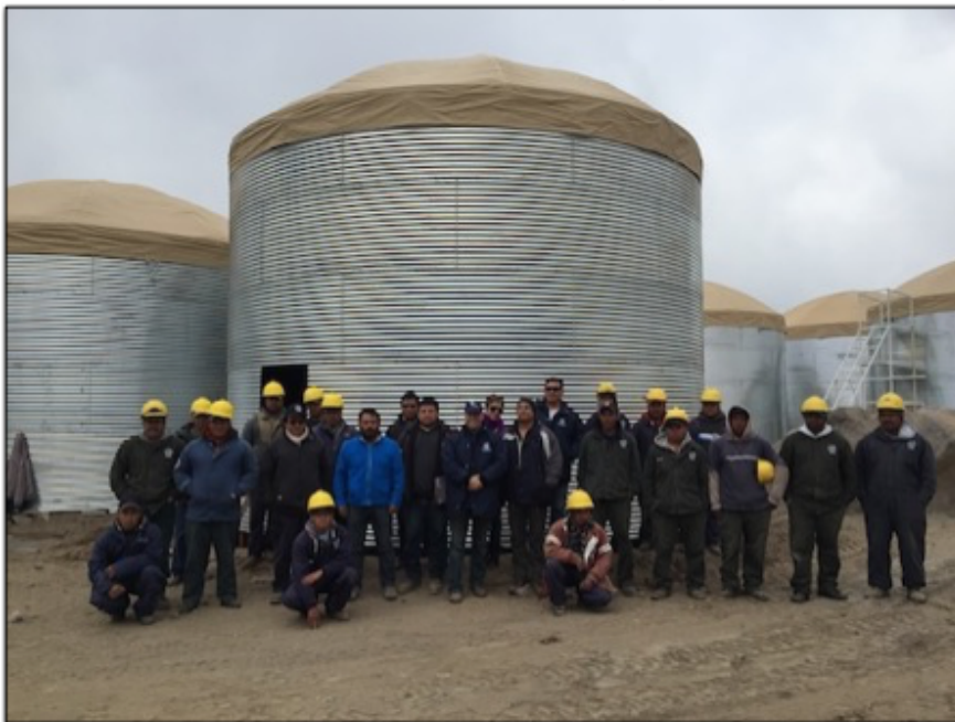
Final tank deployed: December 15, 2014
