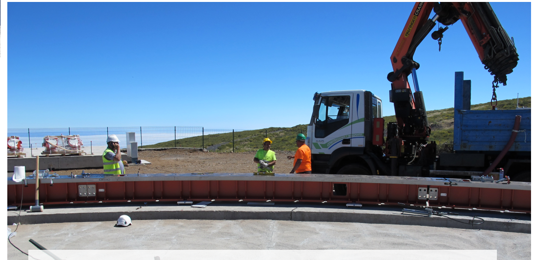
The last segment closed the large circle of the rail system
