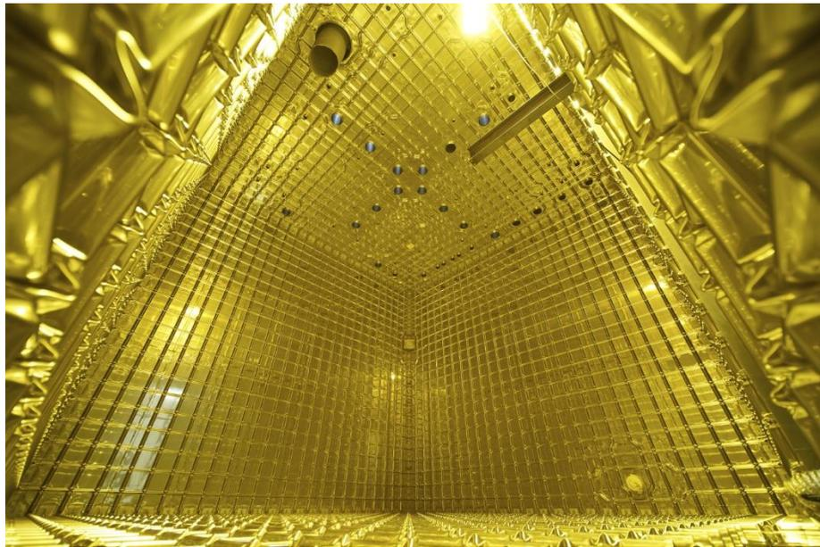
Close collaboration with industry (GTT). Membrane cryostat tech. developed for LNG transport ships
