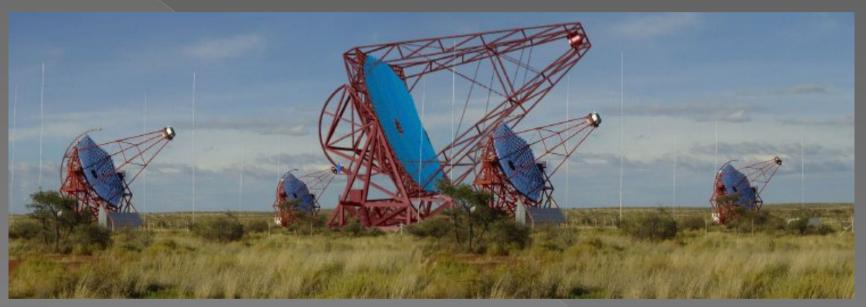
H.E.S.S. II: a very large telescope (28 m diameter) in the centre of the present array (2010) + camera comprising 2048 pixels  $\rightarrow$
