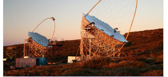
MAGIC (Major Atmospheric Gamma Imaging Cherenkov) - energy range: 50 GeV - 100 TeV - diameter: 17 m - stereo configuration
