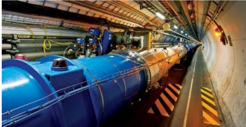
EYETS 2016-2017 : LHC dipole magnet extraction from the tunnel
