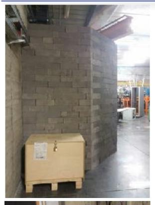
Installed concrete shielding at zero degree line at LNS.
