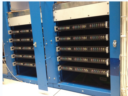
All PP2s installed
