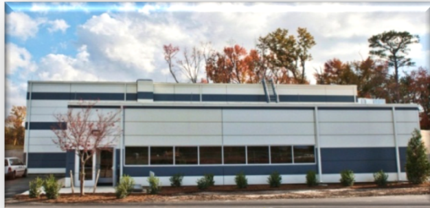
Hall D (new construction)
