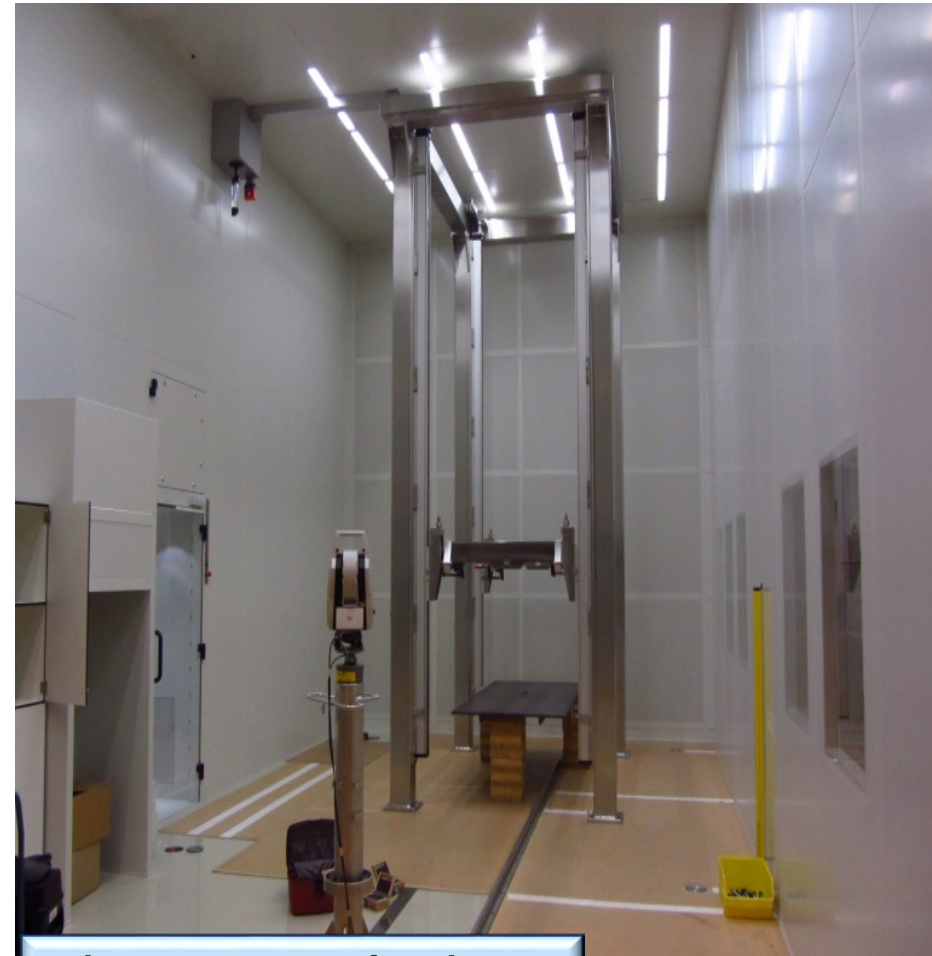
Large structure for clean room (HIE-ISOLDE project)
