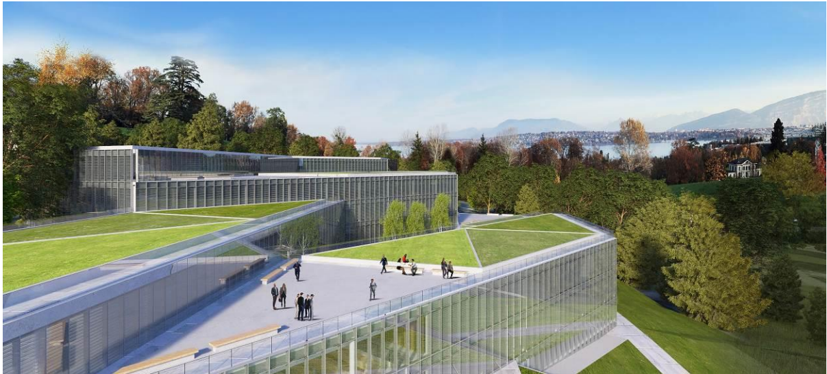
Image 1: New Building H Exterior View from Existing Building E
