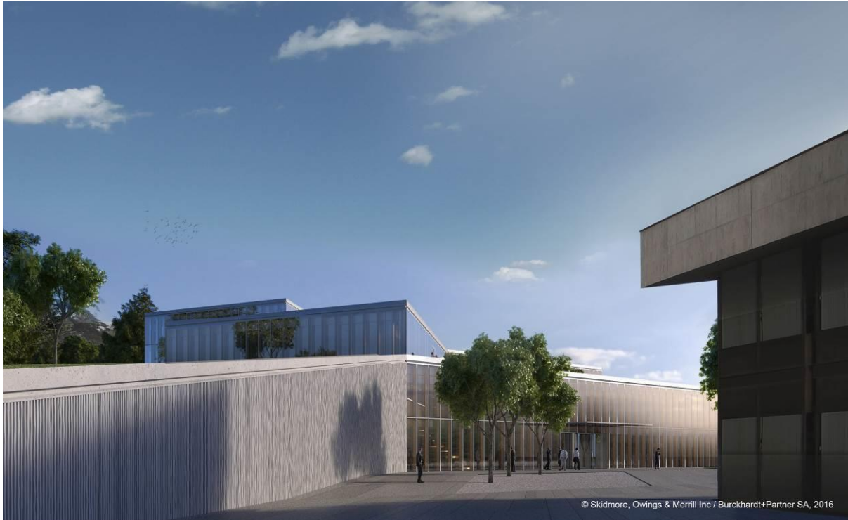
Image 3: New Building H Entrance Level Exterior View from Existing Building E
