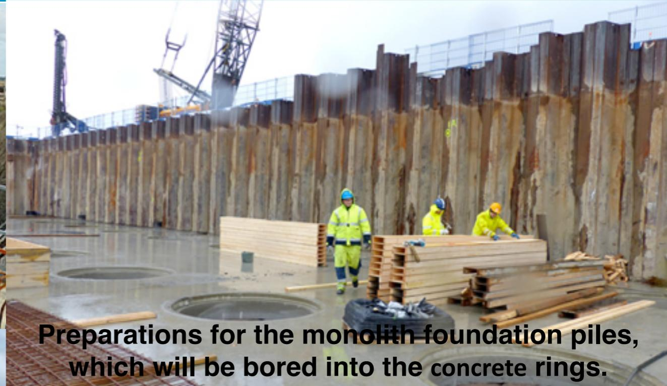
**Preparations for the monolith foundation piles, which will be bored into the concrete rings.**
