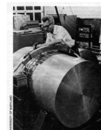
J. Weber Acoustic resonant bar GW detectors
