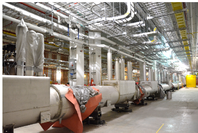
Cryogenic piping installation in the east end of the linac tunnel
