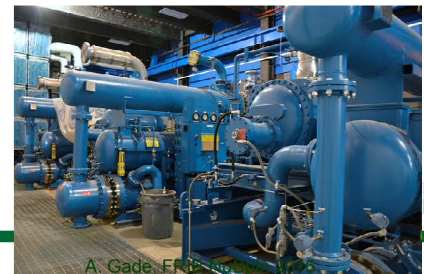
Helium compressors in compressor room
