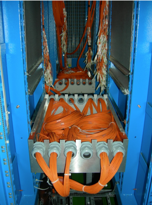
Storage of fibers inside the box
