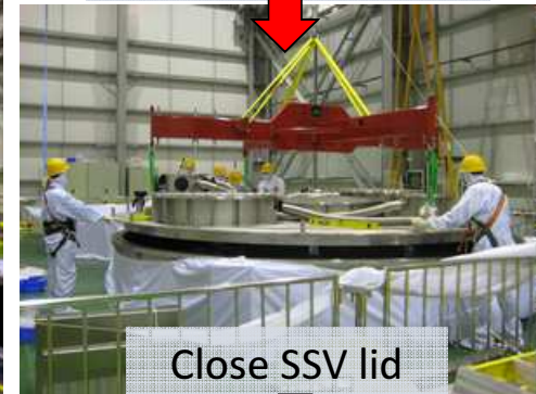
Install top reflector
