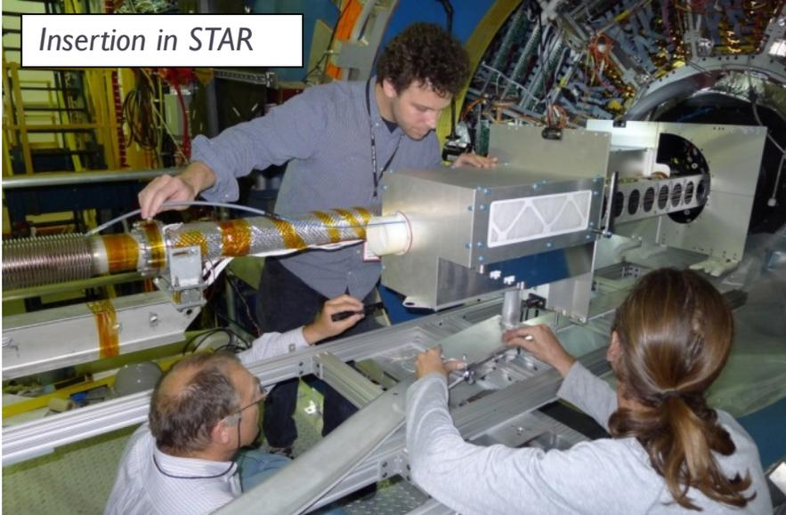
PXL inserted and cabled in STAR
