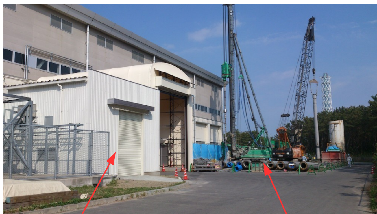
Compressor House (still empty inside)
