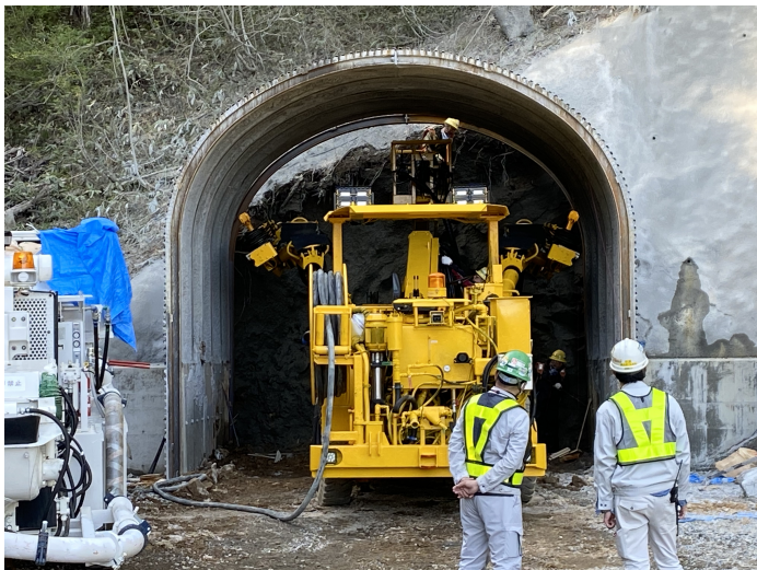
Access tunnel entrance when the excavation just started on May 6, 2021
