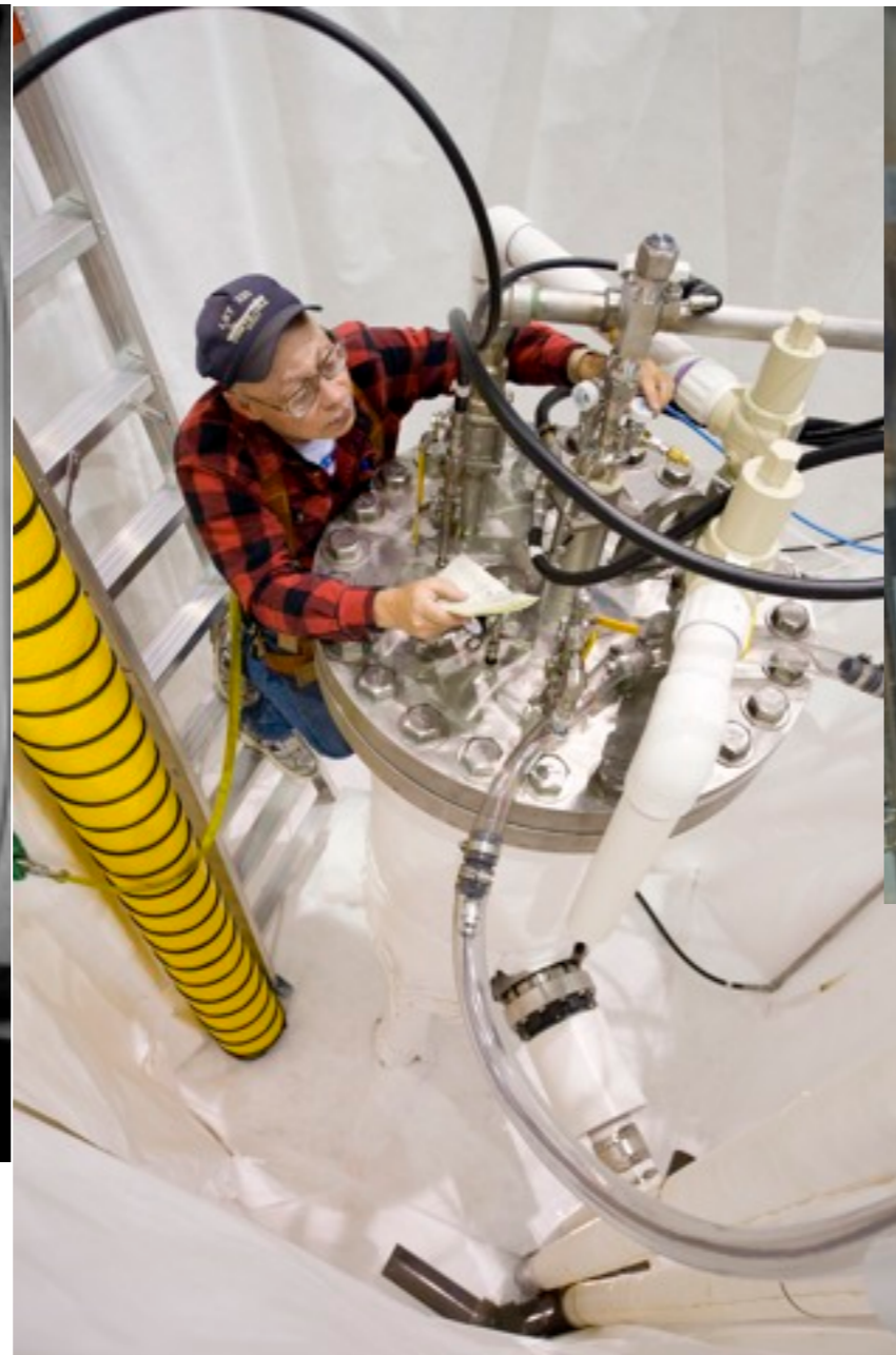
Construction of 60-kg chamber
