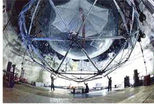
Installing the giant underground tank. But despite its large size the SNO only detects about 10 neutrinos a day.
